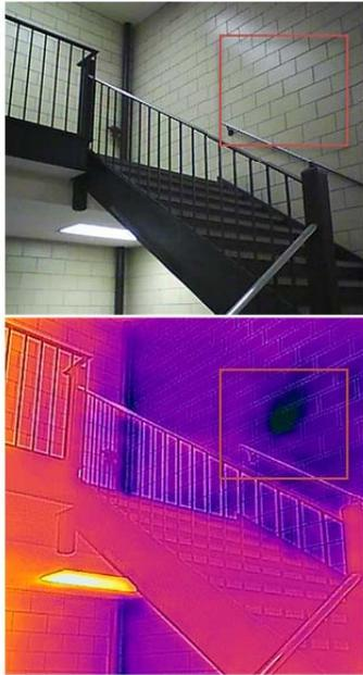
**Figure 5:** A participant in our pilot study surveyed a campus building and noticed an anomalous signature (center of red boxes) in an exterior wall that they could not explain. It was suggested, by other occupants of the building, that this was the site of a previous repair and that perhaps the wall was not restored to its previous condition.
